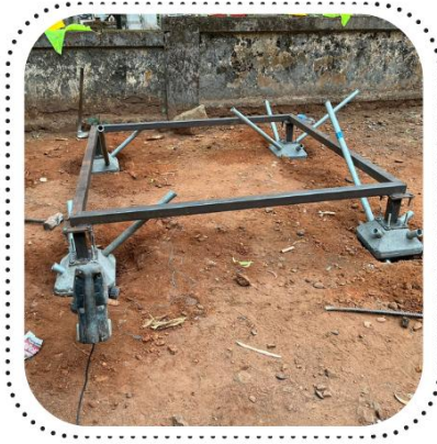
USING THE TIE-BEAM TO JOIN THE ISOLATED NAIL FOOTINGS.
