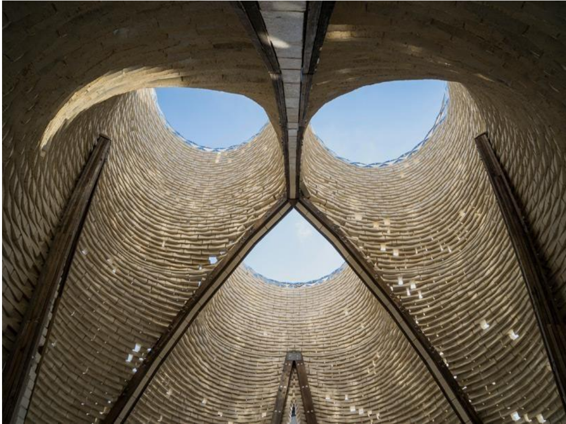
FIG 4.3: Hi-fi by The Living, where the bricks are made of agricultural waste (Courtesy of the living architects)
