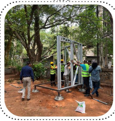
ADJOINING OF THE DEVELOPED FRAMES
