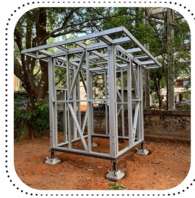
COMPLETED COLD- FORM STRCUTURE
